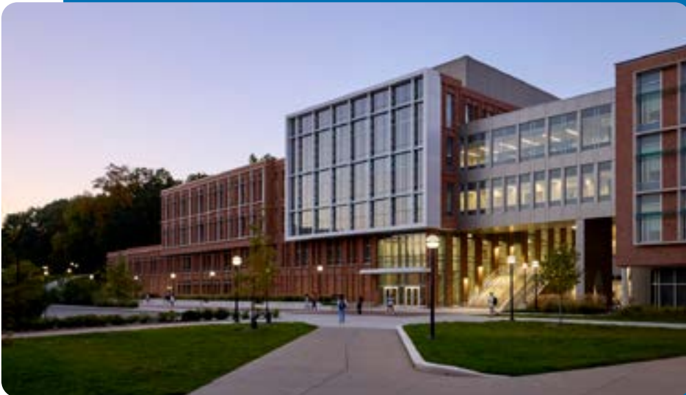
Leinweber Computer Science and Information Building progress
