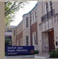
Stanford Lipsey Student Publications renovation
