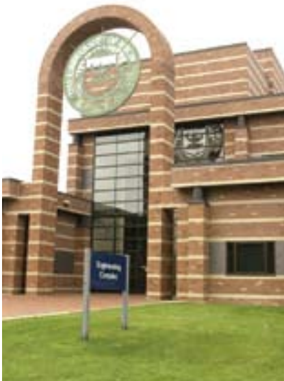
UM-Dearborn Engineering Laboratory Building Expansion and Renovation
