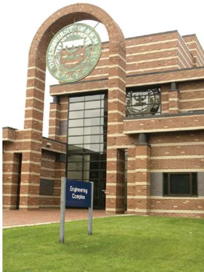
UM-Dearborn Engineering Laboratory Building Expansion and Renovation
